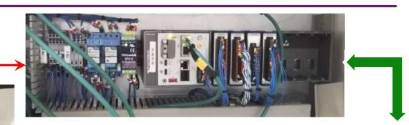
4-20mA and  $\pm$ 10V signals for motion, temperature, generator and power systems currents and voltages, hinge torque, oxygen/hydrogen, vibration, mooring tension, generator and hinge velocity BiSS encoders, overvoltage relays, smoke detectors, earth leakage, bilge pumps control signals, ...
